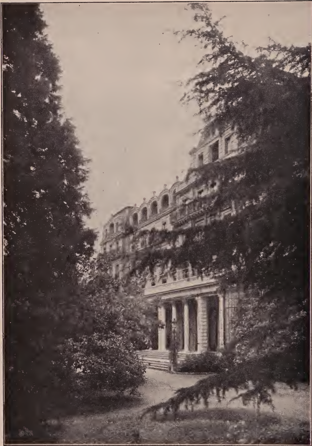
The Palace of the Nations at Geneva, which is only a summer hotel converted into an office building, is in keeping with the moderate expenditures and the sincerity of purpose of the League.
